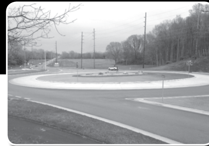
The roundabout at the Hadley Road/CR 700E intersection greatly improved traffic flow in the area.
