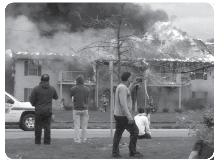
There were two large scale apartment fires in 2013, one at Gladden Farms in April and the other at Stafford Pointe in October. The two fires burned with great intensity and progressed quickly. Firefighters were hurt on both fires due to collapse of the lightweight construction.
