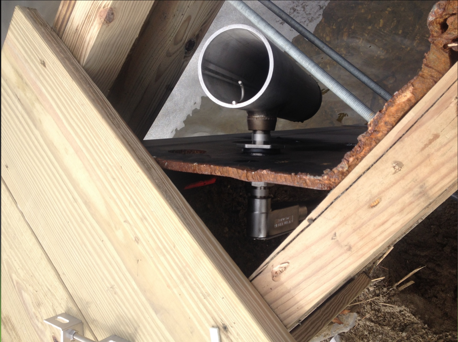
Level Transducer Stilling Tube
