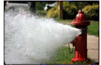
The flushing process is done to remove minerals and sediment that naturally accumulate in water mains over the course of the year. Furthermore, this maintenance allows us to check and record water pressure to ensure the proper operation of the system. Finally, by operating each and every one of the 315 fire hydrants in our water distribution system, we ensure each one is properly maintained and available for use in the event of a fire.
