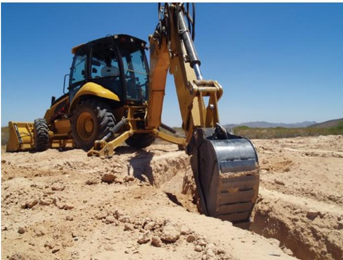
In an instant and without notice, an unsupported trench can give way and a worker can be buried alive. "Even though small amounts of dirt may not seem treacherous, a single cubic yard of dirt can weigh more than 3,000 pounds, which can fatally crush or suffocate workers.
